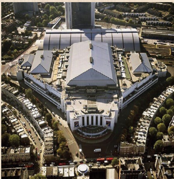
The former exhibition centres (now demolished) were a dominant landmark defining Earl's Court.
